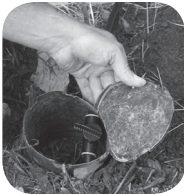
Finished installation of covered valve in planting bed
